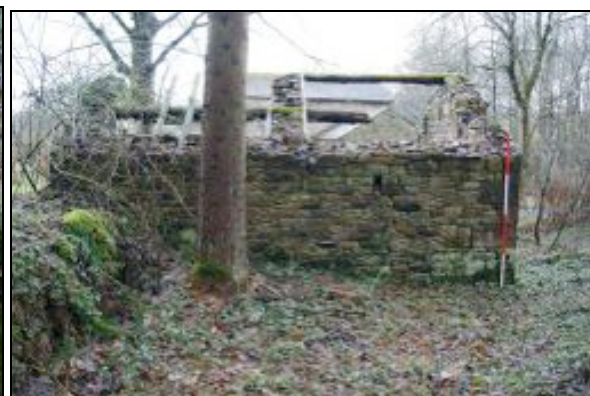
Figure 10. South elevation of pigsty with vents
