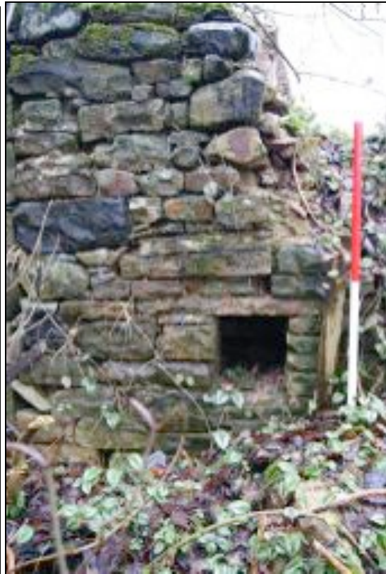
Figure 19. Sluice in additional north wall
