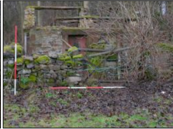
Figure 12. Western elevation showing pens
