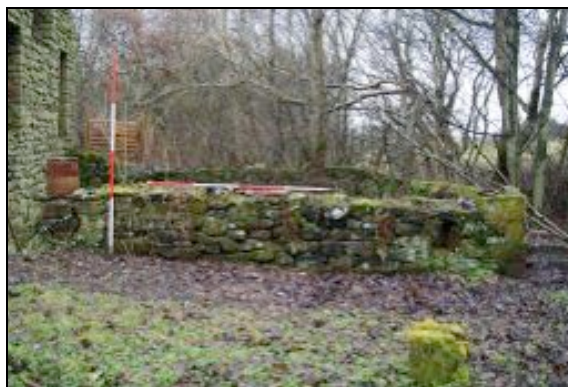
Figure 14. Eastern elevation of ruined mill
