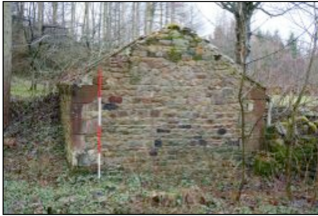
Figure 11. North elevation of pigsty
