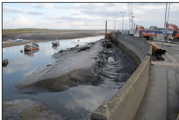
Figure 8. Silt removed western end of Section B
