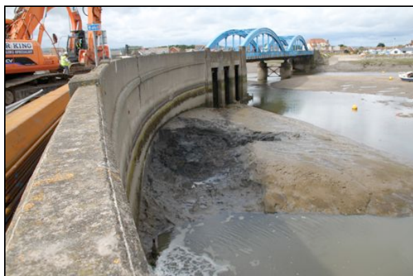
Figure 7. Section A showing excavated silt
