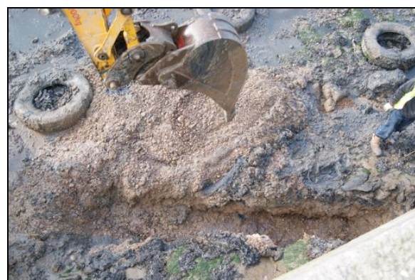
Figure 13. Section D, guide trench with gravel
