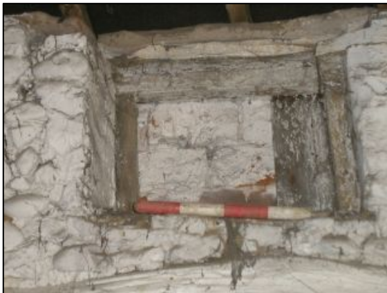
Figures 21 and 22. Filled window and timber lintel above modern door, south wall
