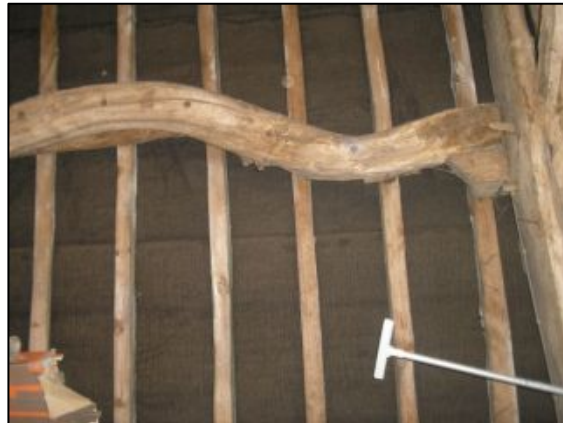
Figures 9 and 10. Roof trusses within Room 2 showing re-used timbers and purlins
