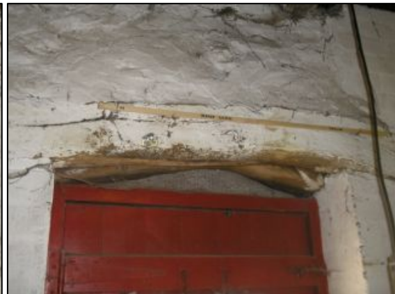
Figures 21 and 22. Filled window and timber lintel above modern door, south wall
