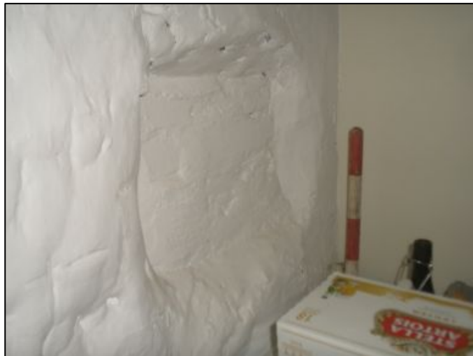
Figures 34 and 35. Recess within clay dabbin wall and view of Room 5
