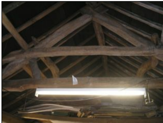
Figures 9 and 10. Roof trusses within Room 2 showing re-used timbers and purlins
