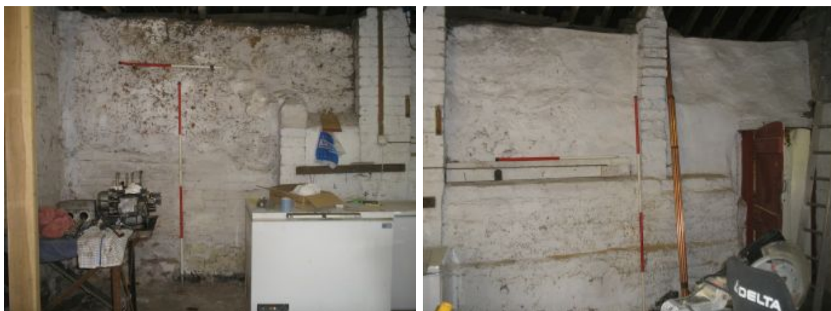
Figures 13 and 14. Western and eastern sections of clay dabbin wall, northern wall
